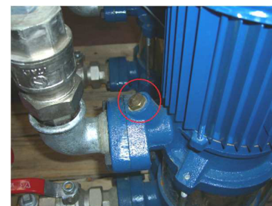
Fig. 7: mounting transducer to venting air hole on the delivery pump
