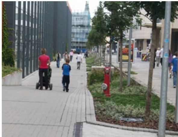
Zilina, Slovakia 5 VAG NOVA 150 Standpost Hydrants
