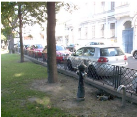
Bratislava, Slovakia 4 VAG NOVA 1885 Standpost Hydrants
