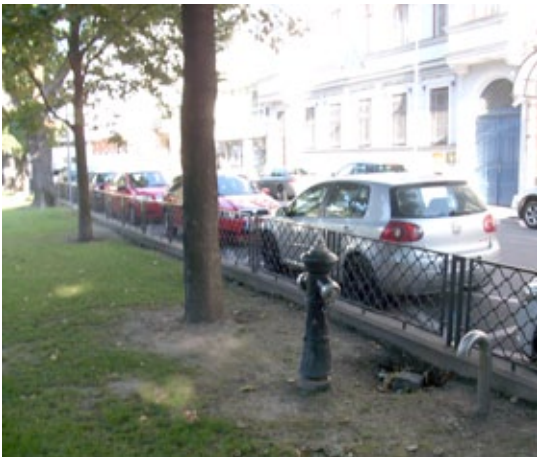
Bratislava, Slovakia 4 VAG NOVA 1885 Standpost Hydrants
